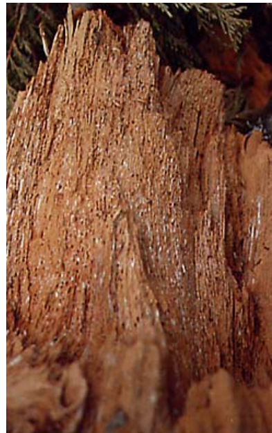
Pitted wood structure common to many white rots
